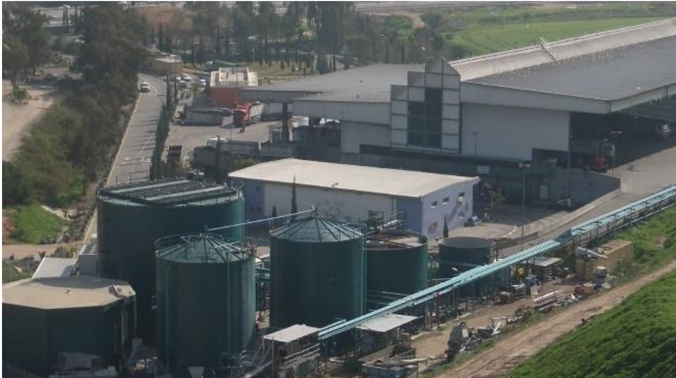
The largest tank is a UASB reactor located near Tel Aviv, Israel
