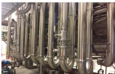
Figure 1: Two banks of 900 gpm for total increase in flow up to 1800 GPM / 2.6 MGD
