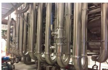
Figure 1: Two banks of 900 gpm for total increase in flow up to 1800 GPM / 2.6 MGD
