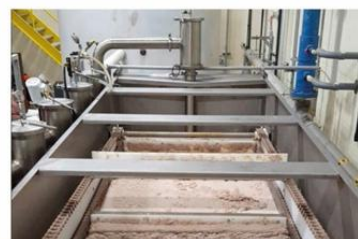
Figure 1: Two banks of 900 gpm for total increase in flow up to 1800 GPM / 2.6 MGD
